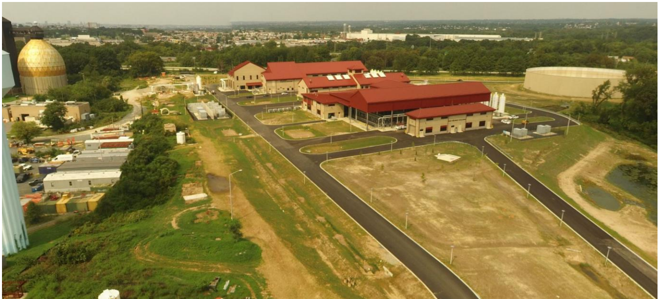
Back River WWTP Headworks Project – Landscaping; September 2021
