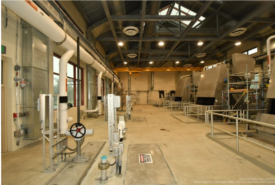
Back River WWTP Headworks Project –Fine Screen Facility; September 2021
