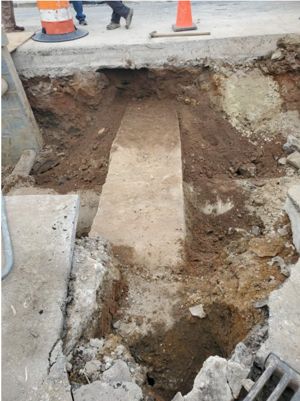
Figure 3-6: SC 941 – 18" Encased storm drain in path of new 48in. PCCP Sewer
