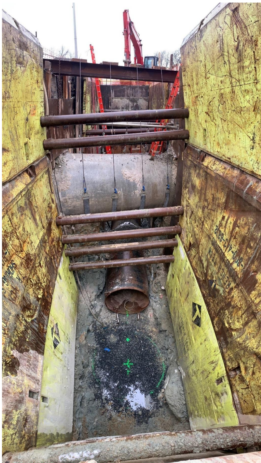
Figure 3-5: SC 940 – 42in. Open-Cut under 66in Water Main at 2800 N Dukeland Street
