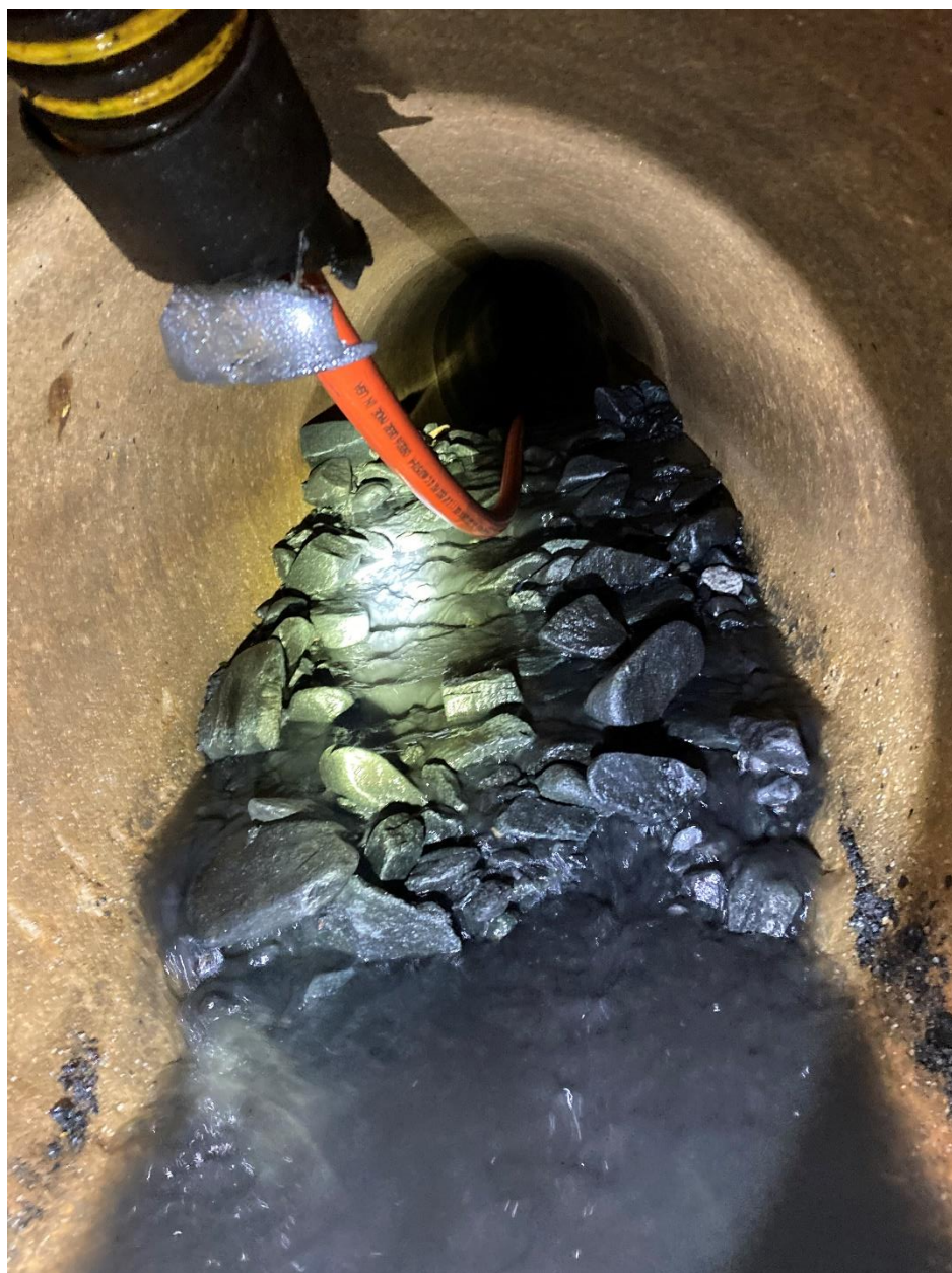
Figure 3-11: SC 977 – Heavy debris clogging sewers (Picture 2 of 3)
