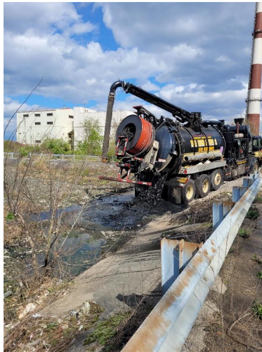
Figure 2-3: Material that is being extracted from interceptors is de-watered at a holding pond and transported to the City's Quarantine Road Landfill
