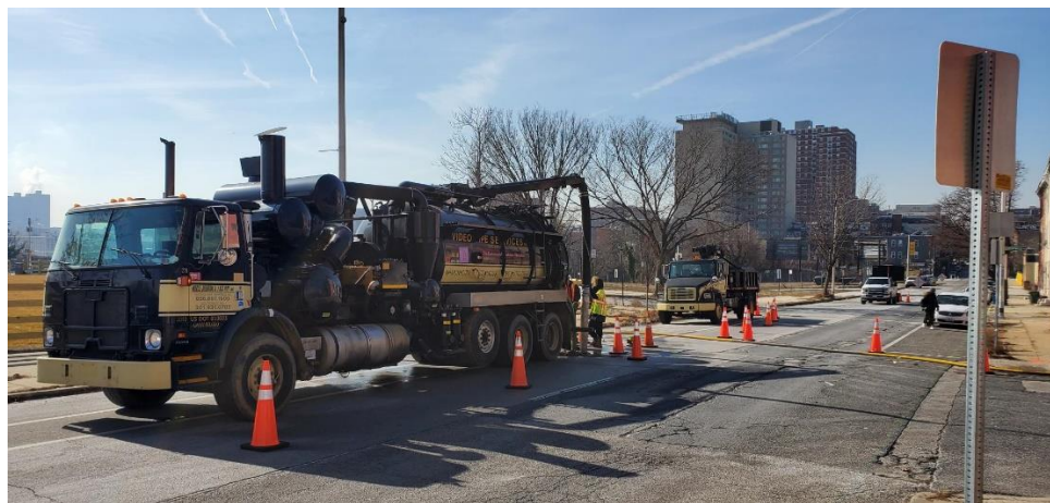
Figure 2-2: Material that is being extracted from interceptors is de-watered at a holding pond and transported to the City's Quarantine Road Landfill
