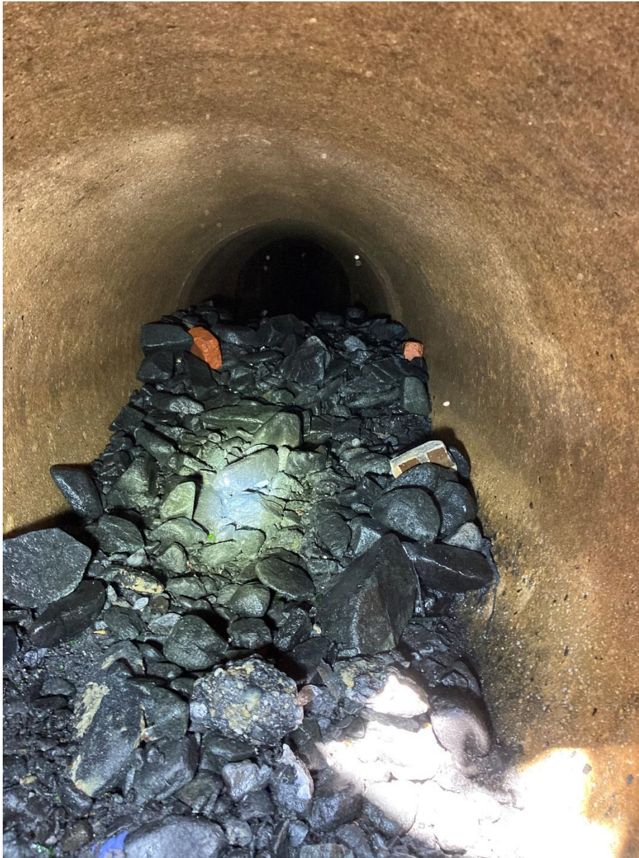
Figure 3-10: SC 977 – Heavy debris clogging sewers (Picture 1 of 3)
