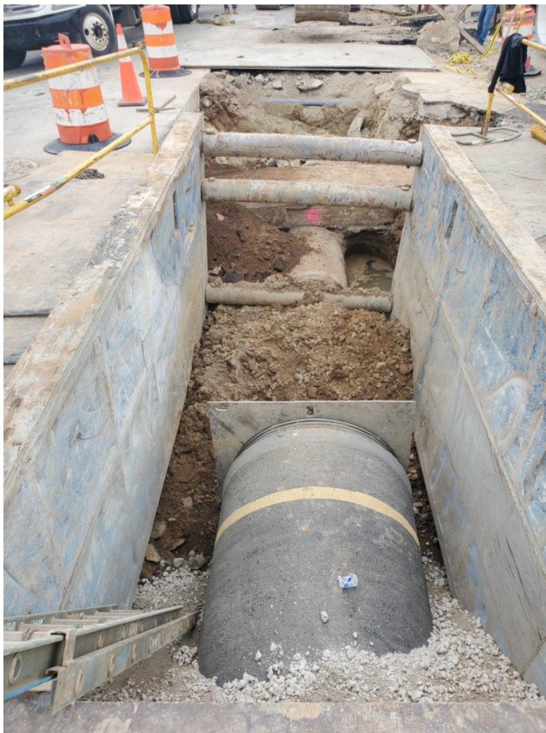
Figure 3-7: SC 941 – PCCP Sewer installation
