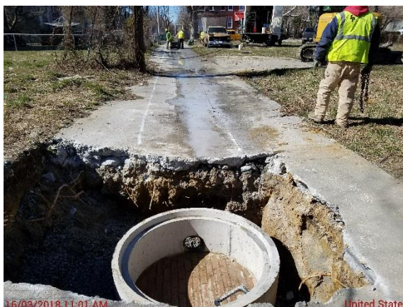
SC 953 New manhole installation
