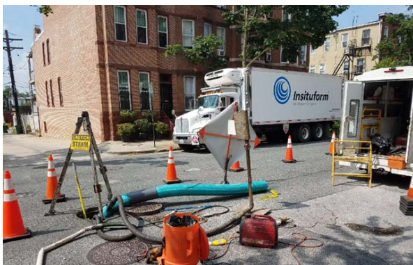
SC 976 progress photo
