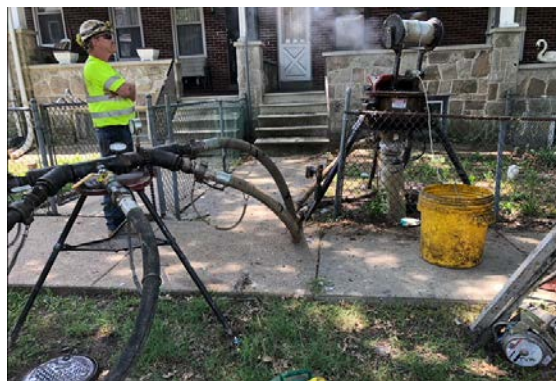
SC 976 progress photo
