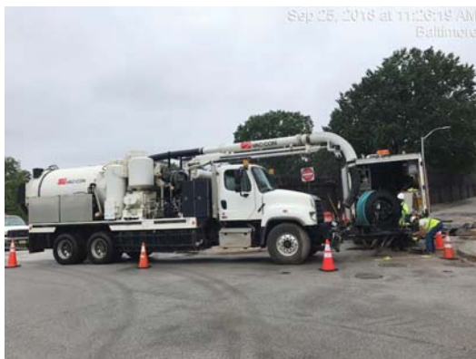
SC 963 progress photo
