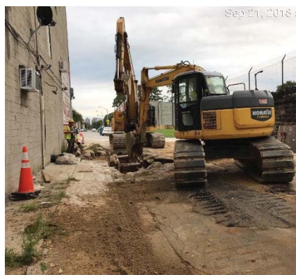
SC 963 progress photo
