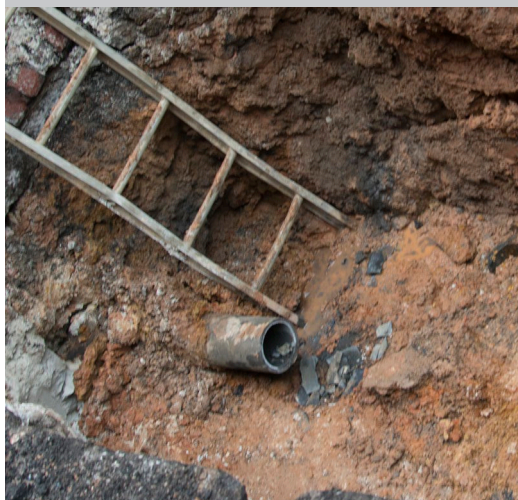
Below: A water main repair in process.
